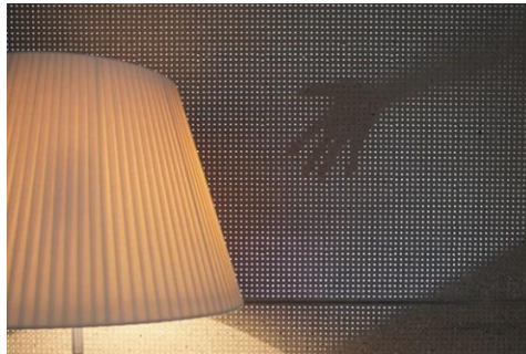
Figure 7 the application of transparent concrete panels in form of a partition wall in “Europe Point”
